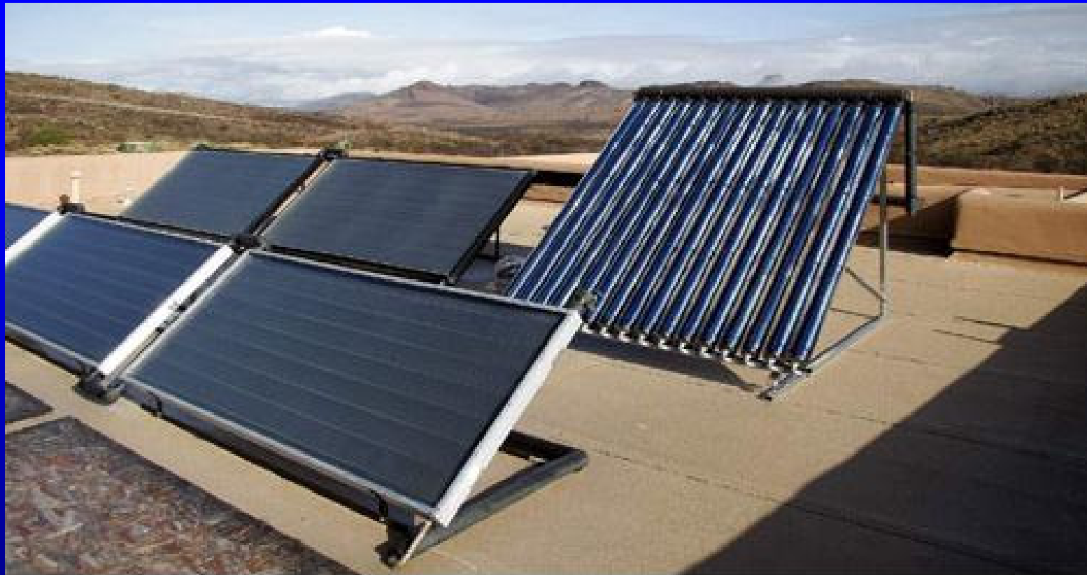
A combination flat plate/evacuated tube solar installation.
